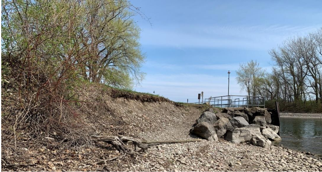
Figure 14 – Area of erosion south of existing sheet pile wall (03 MAY 2021)
